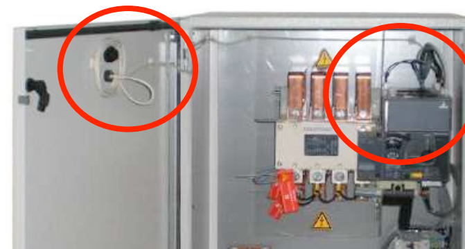
RJ45 PORT for ATyS D10 connection
